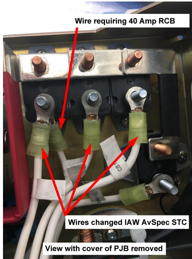
FIGURE 3 – OEM Circuit Breaker Installation
